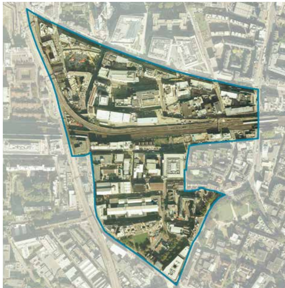
Figure 45: Bankside Commercial - Aerial Overview
