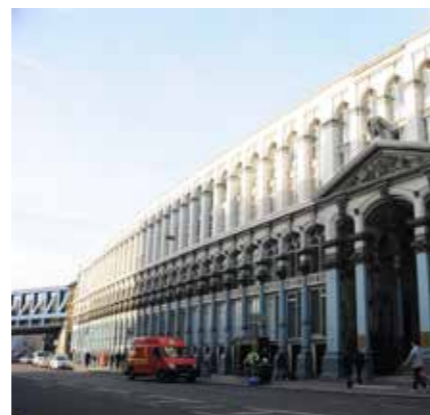
The Hop Exchange, Southwark Street
