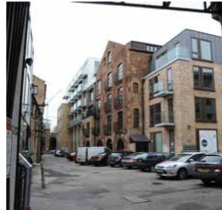
Views into internal block space
