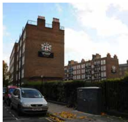
Local Authority Housing
