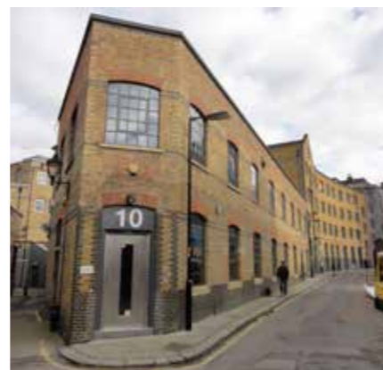
Converted warehouses, Valentine Place
