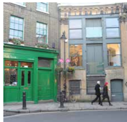
Shops and converted warehouses, Park Street
