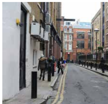
Converted warehouse south of Tooley Street
